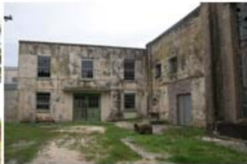
old water plant.jpg
